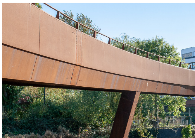
Active Travel Bridge in Northampton
